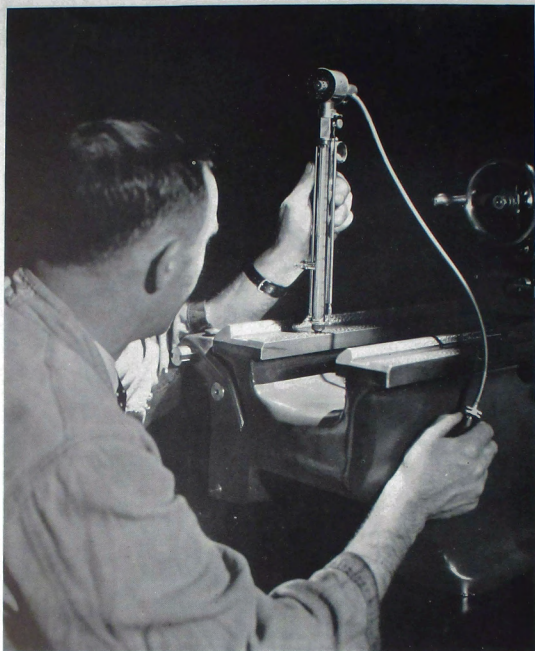
TESTING THE HARDNESS OF A MONARCH LATHE BED
