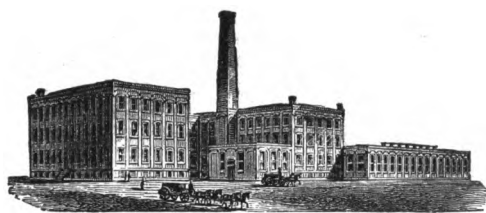
REAR VIEW OF NO. 1 BUILDING.
