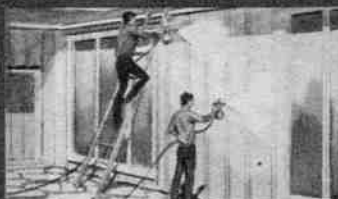
Power-spray paint... even operate two guns at once
