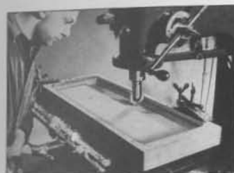
The machine is exceptionally useful for panel sinking operations as shown above.
