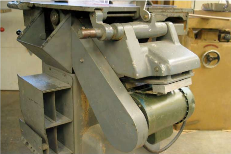
Figure 50 side view of the new motor installation.
