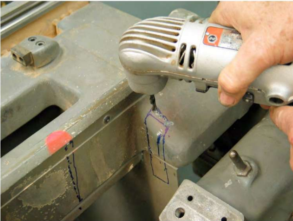
Figure 245 Drill a line of holes that are very close together.
