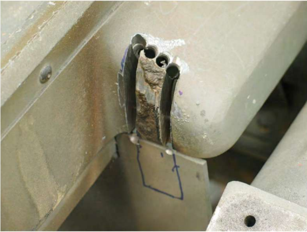
Figure 278 Slot s are not cut and the opening is ready for removal.
