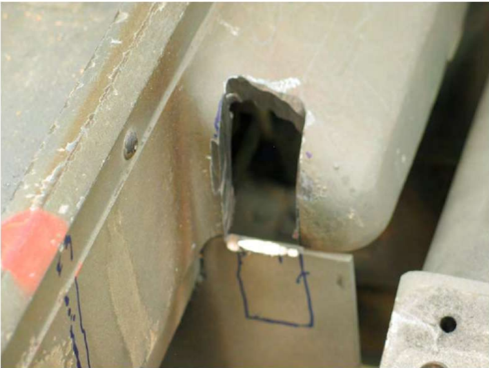
Figure 291 Opening complete and now the bottom area will be ground out.
