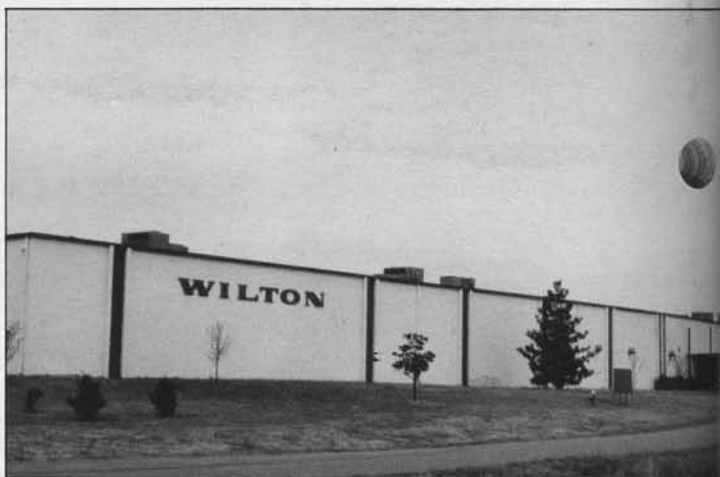
Plant at Winchester, TN
