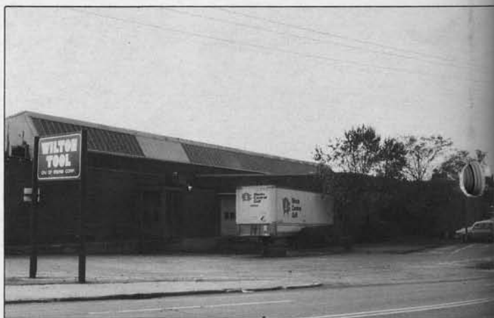
Plant at Schiller Park, IL
